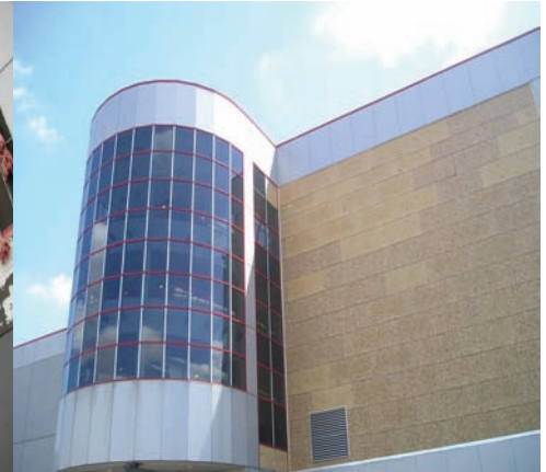
Board up completed by G.S. Jones
