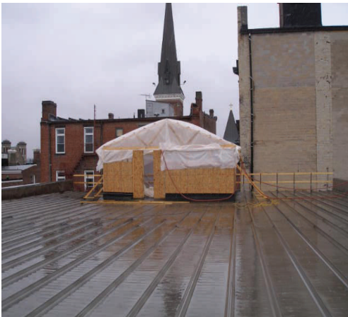
Temporary enclosure over damaged roof
