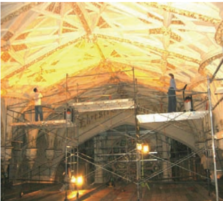
Rolling scaffold to reach domed 56 ft ceiling
