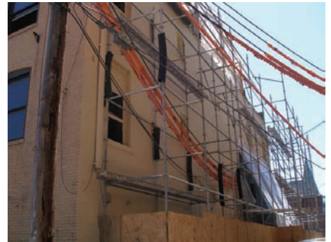
Scaffold system around high voltage lines.
