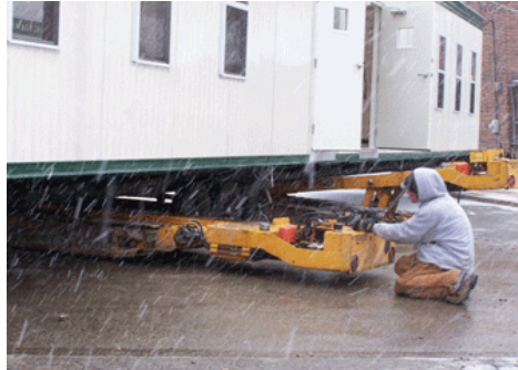
Workers position equipment to move modular classrooms
